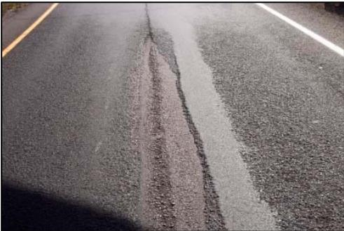
**SHOVING:** Lateral displacement of paving material due to traffic, generally resulting in the bulging of the surface. It is caused by lack of stability in the subgrade, base, or surface layers. It requires the removal of the affected area followed by deep patching with asphalt. *Photo courtesy of FHWA.*
