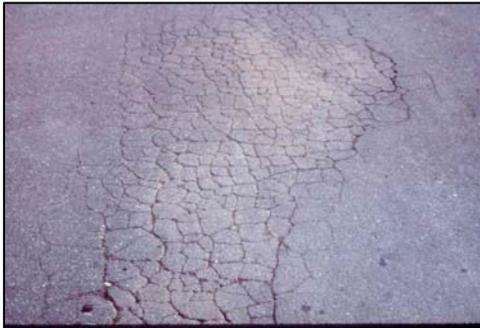
**SHRINKAGE CRACKS:** Interconnected cracks forming a series of large polygons, usually having sharp angles at the corners. Shrinkage cracks are not related to traffic loading. It is caused by volume change in the base or subgrade. It requires monitoring of the hairline cracks, crack sealing, or fog treatment with asphalt material possibly followed by a surface treatment over the entire surface. *Photo courtesy of MnDOT.*
