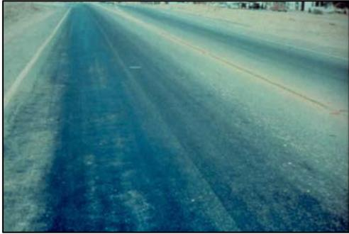
**POLISHED AGGREGATE:** Aggregates in the surface of the pavement that have been polished smooth. It is caused by naturally smooth, non-crushed gravels and/or crushed rock that wears down quickly under action of traffic. It requires covering the surface with a asphalt pavement treatment that has good frictional characteristics. *Photo courtesy of US DOT.*
