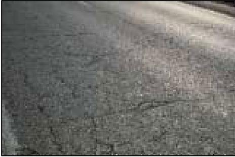
**ALLIGATOR CRACKING:** Interconnected cracks forming a series of small polygons, the pattern resembles an alligator's skin, and is a load-related structural distress found in the wheel path. It is caused by excessive deflection of the surface over unstable pavement base or subgrade layers that leads to fatigue failure. The unstable support usually is the result of saturated layer or layers or an unstable pavement design. It requires deep patching with asphalt.
